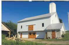
Evans Barn After
